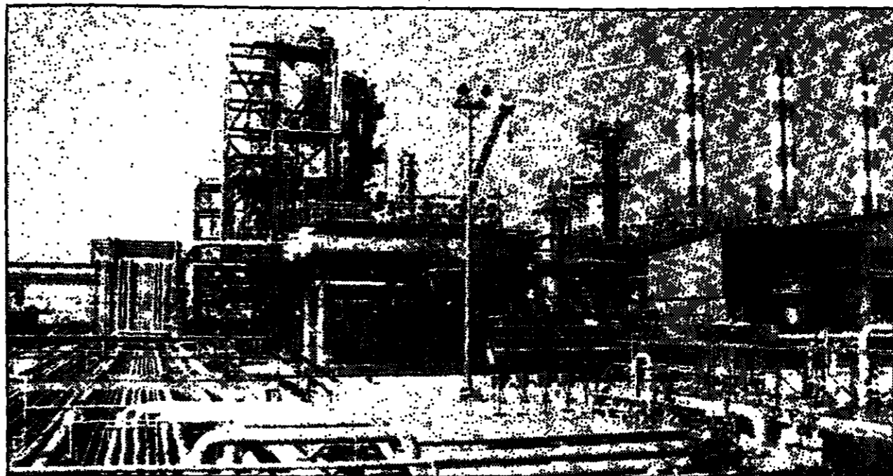
Petrokem's new butene-1 plant began operations this fall in Al-Jubail.
